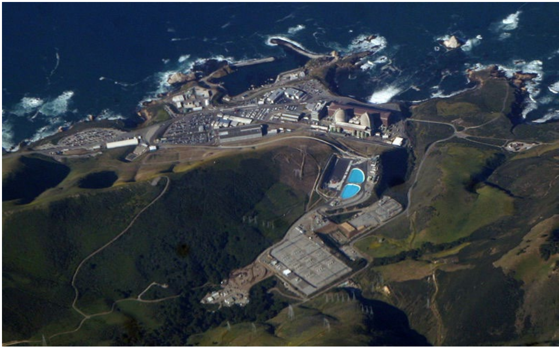
Diablo Canyon Power Plant , on the coast of California.(image credit Doc Searls)
