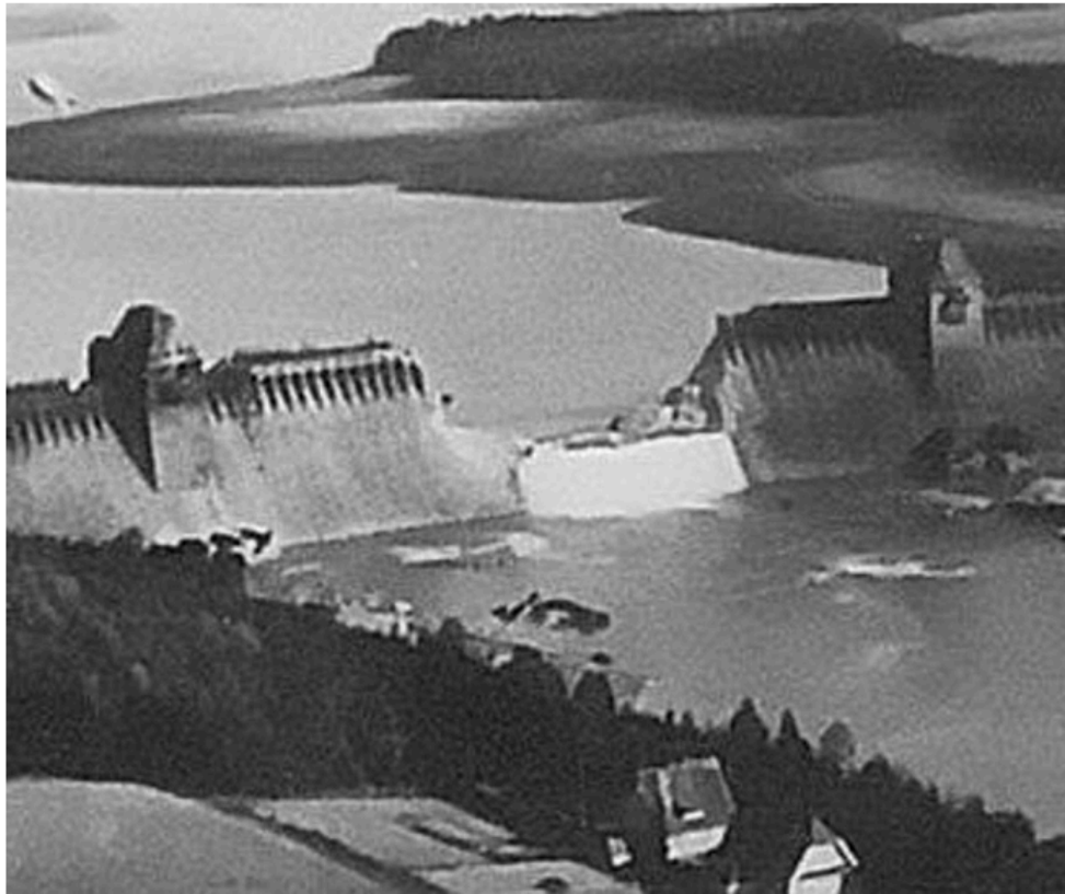
Figure 3. The Banqiao Dam after the collapse. The exposed shoreline in upper part of scene gives a feel for the total release of water.
