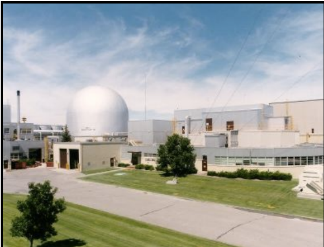
Figure 1. The Experimental Breeder Reactor (EBR-II) at its test site at the Idaho Argonne National Lab West now known as the Idaho National Lab. The EBR-II ran for 30 years and as an IFR the last ten years. On April 3, 1986, two tests demonstrated the inherent safety of the IFR concept. These tests simulated accidents involving loss of coolant flow. Even with its normal
