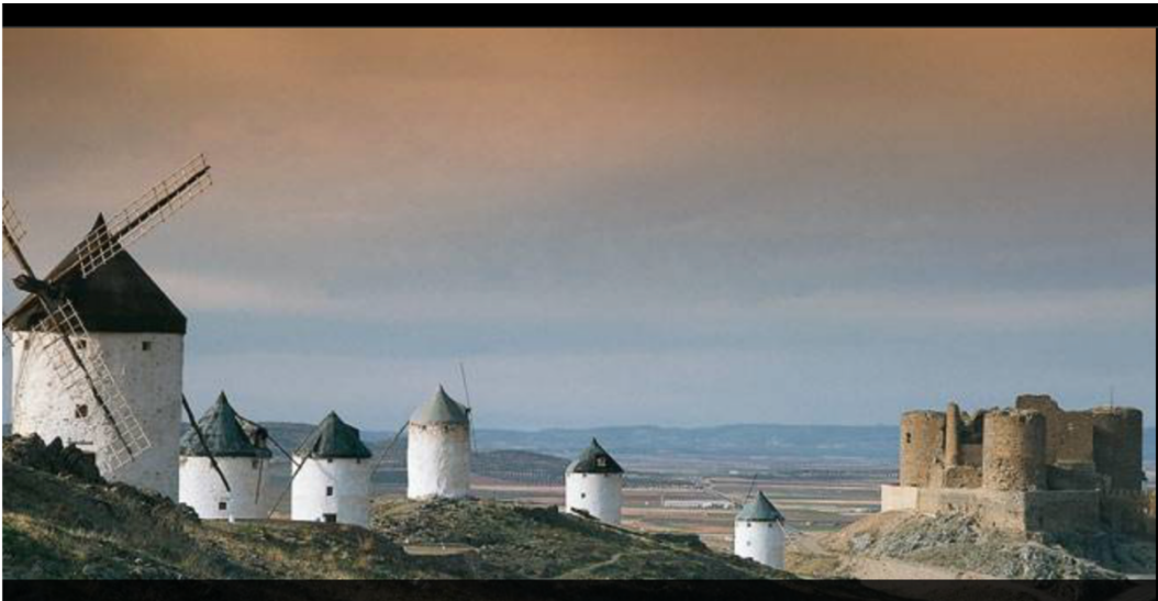
Figure 5. Six of the 12 historic windmills of a 17 th century windfarm in Consuegra, Spain. A medieval castle is in the background. Each windmill was manually turned to face the wind. 70-pound bags of grain were poured from the top of the windmill into a grinding wheel below.
