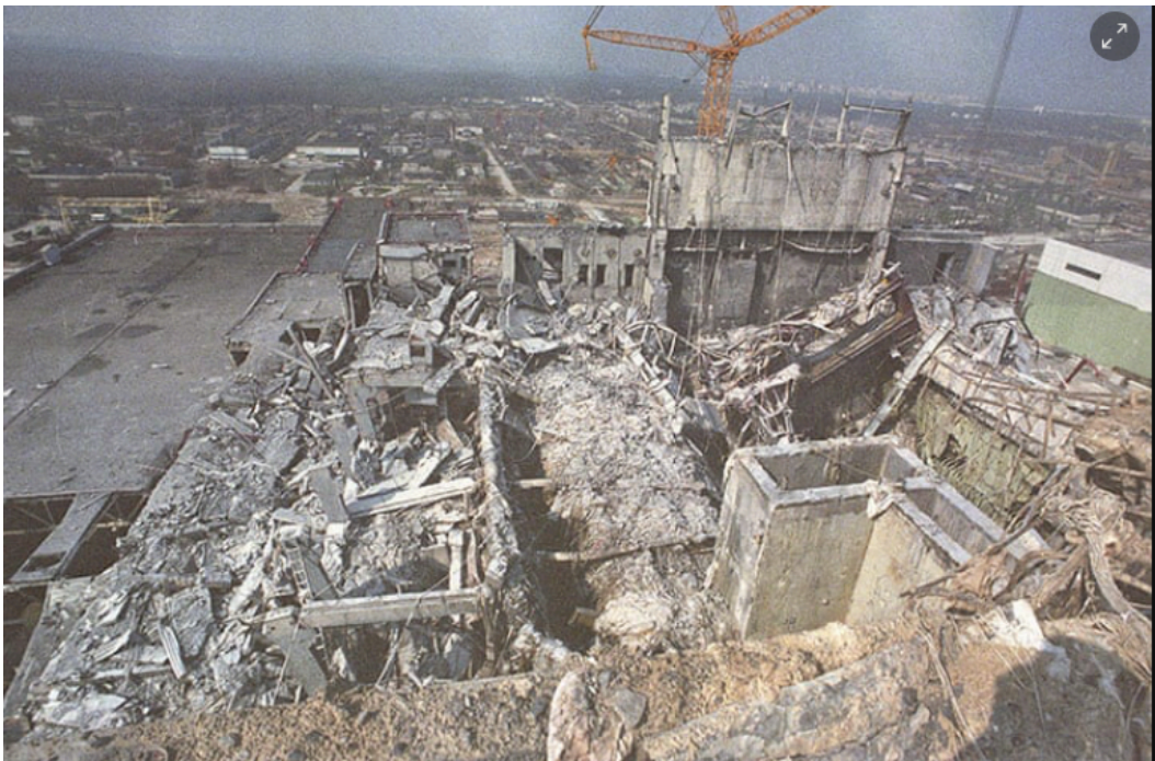
Figure 3. The remains of Chernobyl reactor number-4, from the roof of the third reactor.
