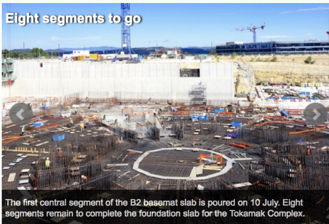
Figure 2. The fusion reactor construction in Cadarache, France.
