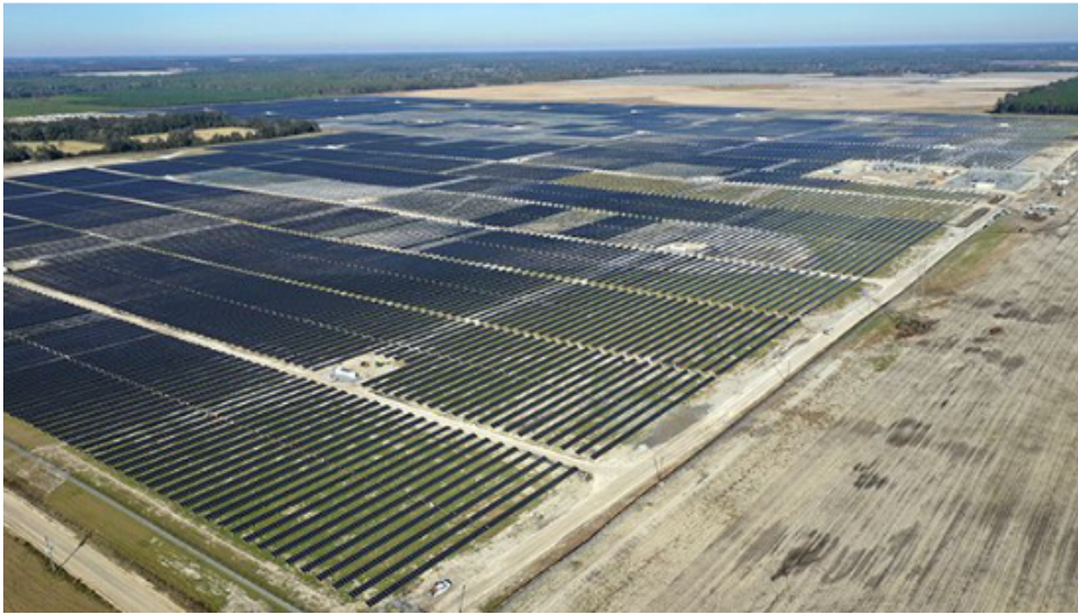
Figure 4. An 80 MW medium-scale solar farm in Jasper, Florida. The shadow over the PCs is believed to be a cloud.
