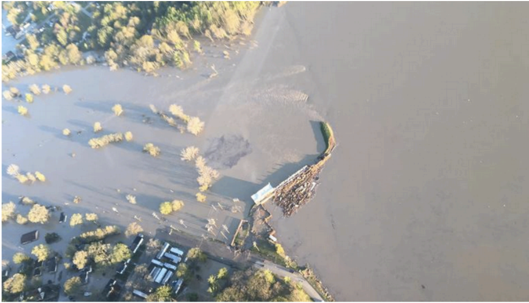
Sanford Dam in Midland County breached. (photo by Martin Szeliga)
