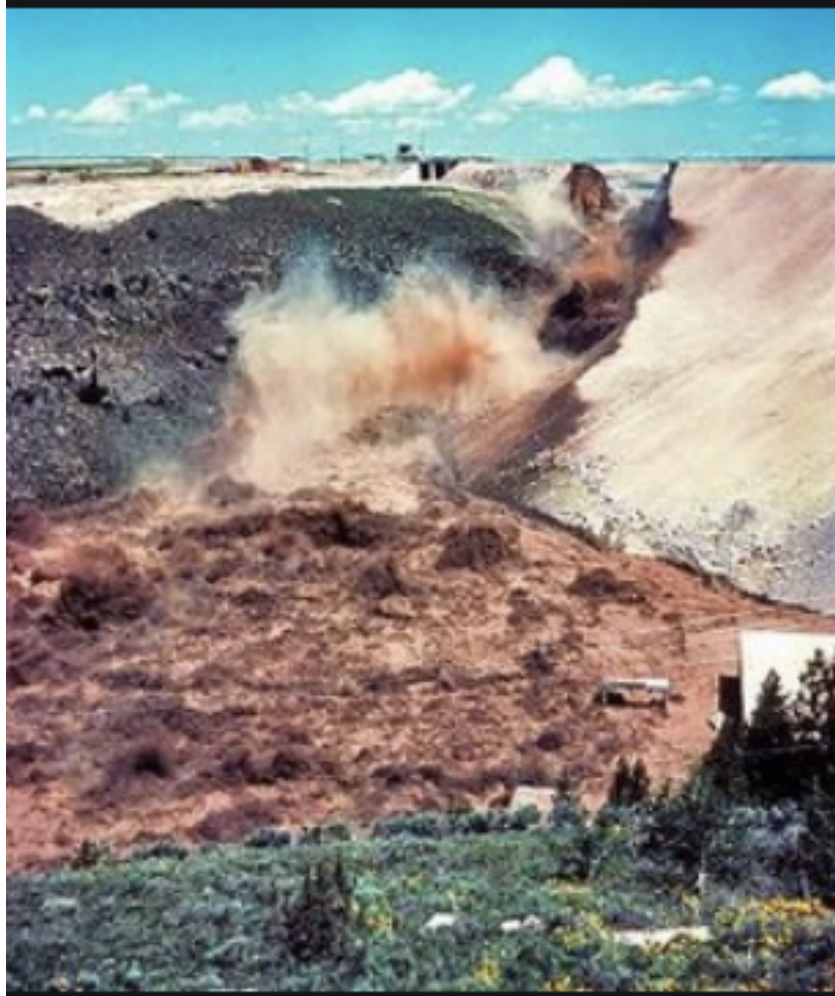
Figure 6. Photos showing initial rush of flood water from the Teton Dam. ( Damfailures.org , en.wikipedia.org )
