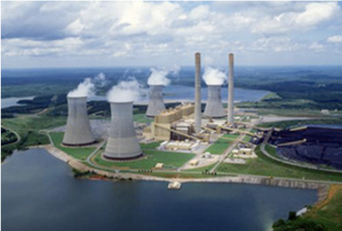
Figure 1. Robert Scherer Power Plant emits 27 million tons of CO 2 per year. It has four units that can deliver a total nameplate power of 3.5 GW with a capacity factor of about 61%. [Photo courtesy of Georgia Power].
