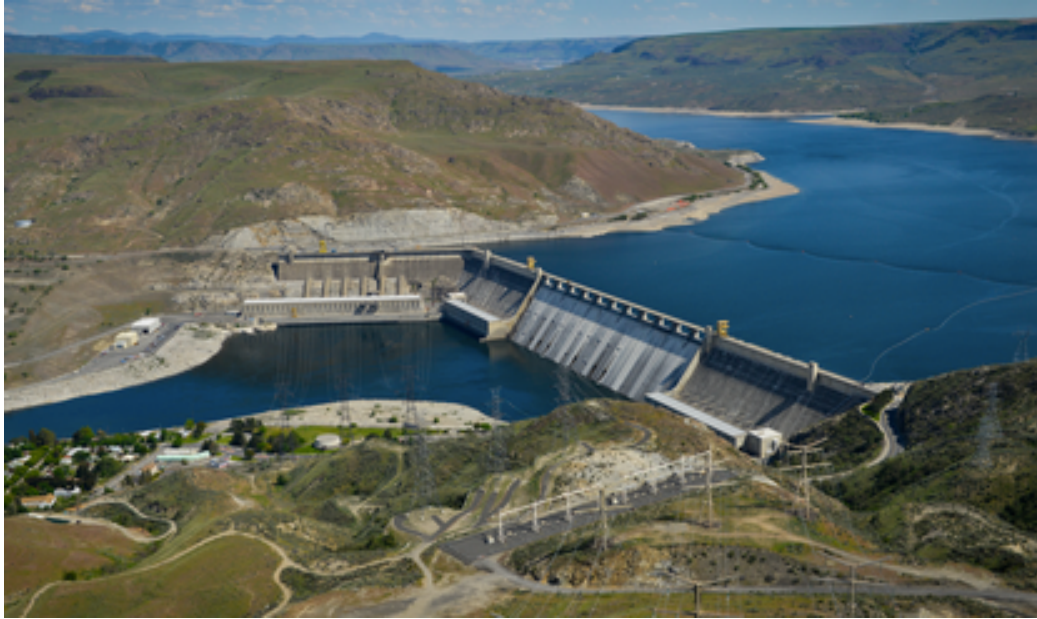
Figure 1. The Grand Coulee Dam in Washington state, the deep canyon reservoir is part of the Columbia River. The dam has a water height of 380 feet, a nameplate of 7.1 GW, a capacity factor of 36% and a yearly output of 20.24 tWh (usbr.gov).
