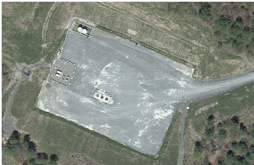
Figure 1. (a) Truck and other equipment complexity at a single drill site. The work goes on 24 hours per day, seven days per week. (Photo from
